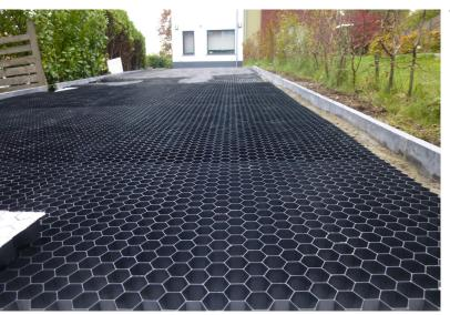
**The Gravel Stabiliszation** range is designed to ensure a stable, sustainable and navigable gravel surface.
